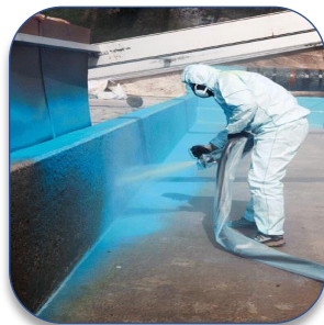
Water Proofing Works
